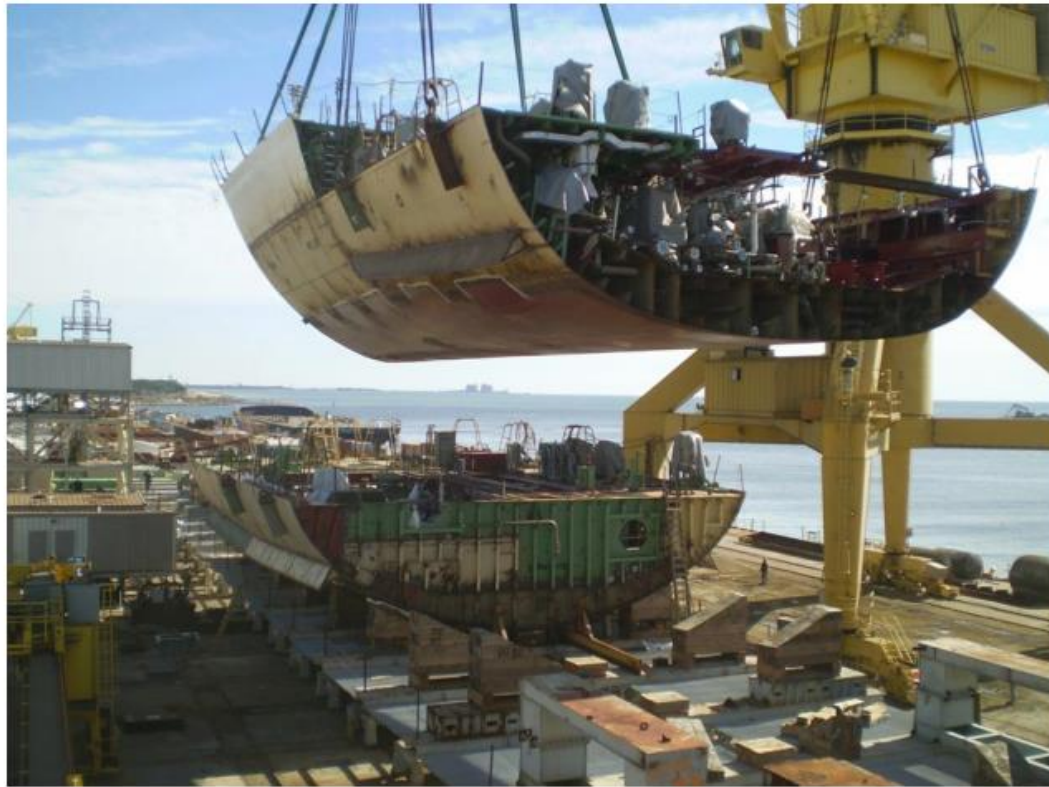
The first grand blocks of the future USS John Finn (DDG 113) are erected on the building ways at the Ingalls Shipbuilding yard in Pascagoula, Miss. Huntington Ingalls Industries photo.
