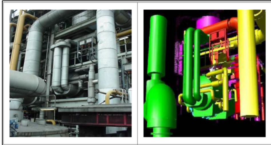
Figure 10. 3D Model of Industrial Piping (Quintero et al., 2008)
