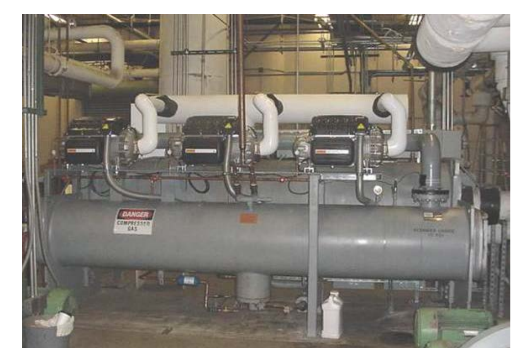
Magnetic Bearing Chiller Compressor Installation at NRSW San Diego, CA
