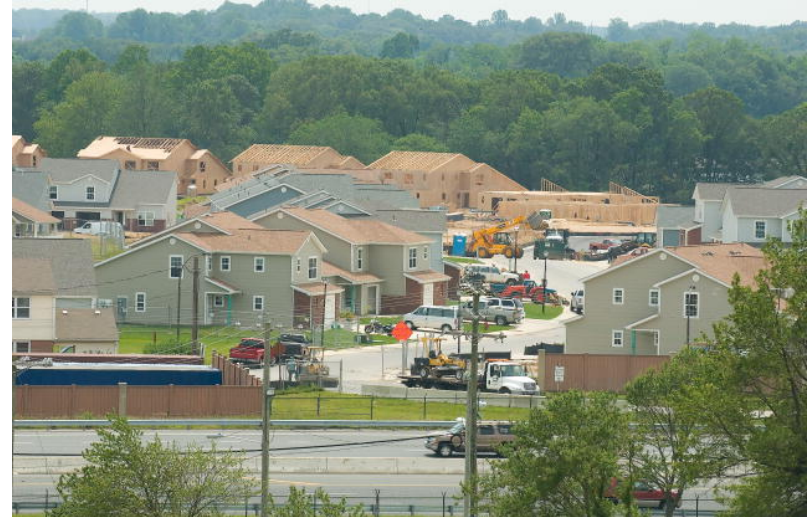
A long shot view of a housing area just outside Dover Air Force Base, Del., June 4, 2008, as seen from atop the 436th Civil Engineering Squadron heat plant building.
