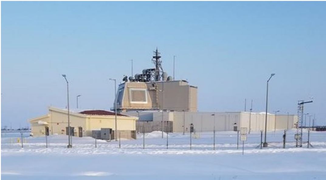
Figure 4. U.S. Aegis Ashore Missile Defense System in Romania. Source: U.S. Aegis Ashore Missile Defense System Romania (2023)
