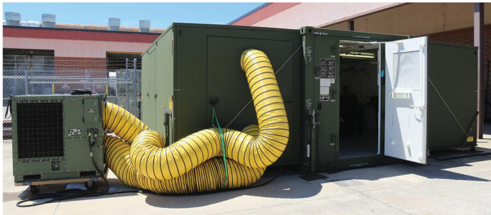
Figure 1. XFAB in Deployed/Operating Configuration. Note Environmental Control Equipment Connected to XFAB. Source: Roach (2021).
