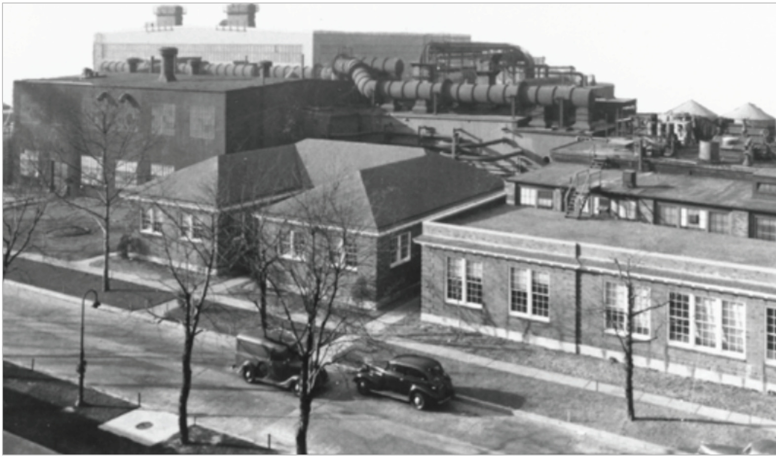
Naval Boiler and Turbine Laboratory in 1943. Source: Naval Surface Warfare Center Philadelphia Division Public Affairs, 2016.
