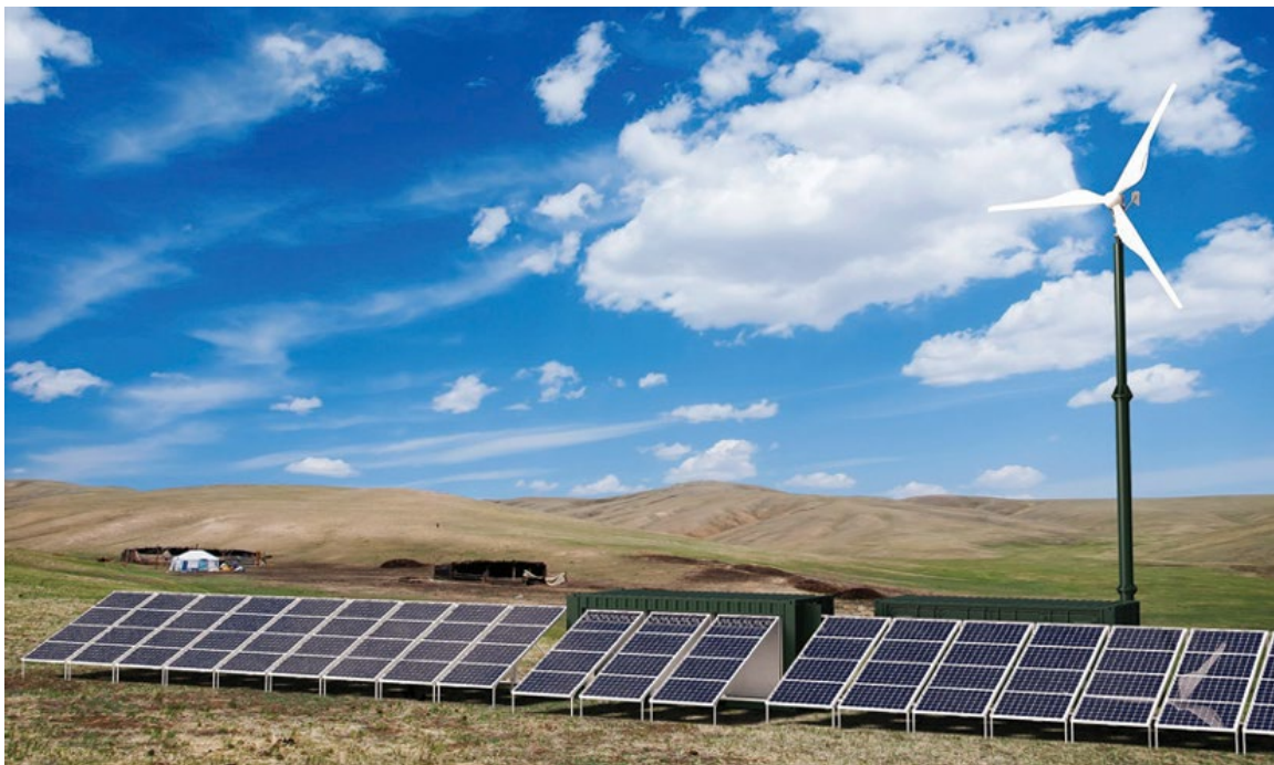
Figure 4. Hybrid Power Generation System (HPGS) demonstration figure. Source: Gogoreliani et al. (2021, p.29). HPGS includes PV and wind production, along with two containers. One container includes two generators, an energy storage system, and an automation system; the other container stores PV-cells.
